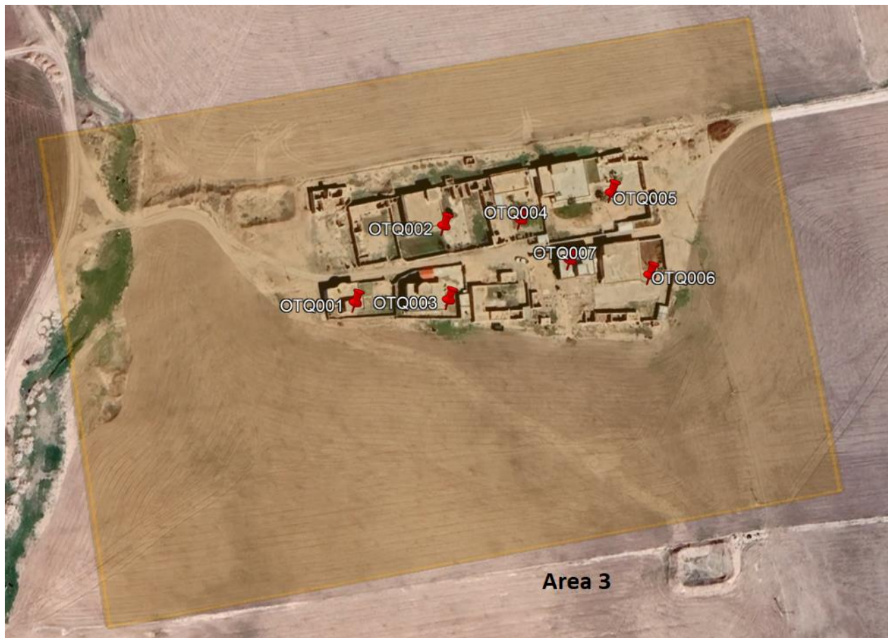
Figure 4 Area 3, Contains 7 Houses to be rehabilitated in Old Tel Qasab Village
