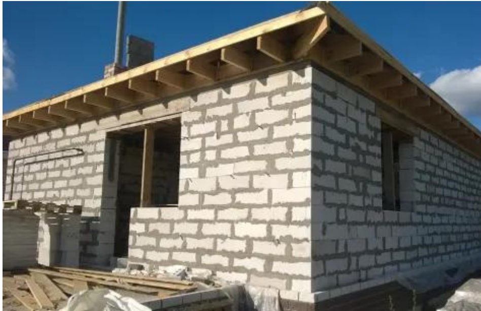
Fig.3.3 Construction of house using Concrete Block Masonry.
